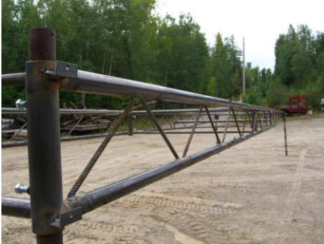
Dock Frame – Unpainted Truss Detail
