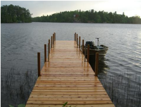
New Cedar Decking On An Eagle Dock
