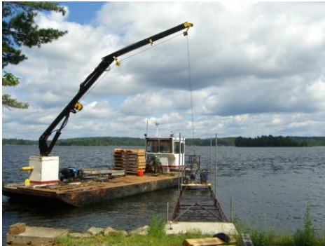
New Dock Installation!
